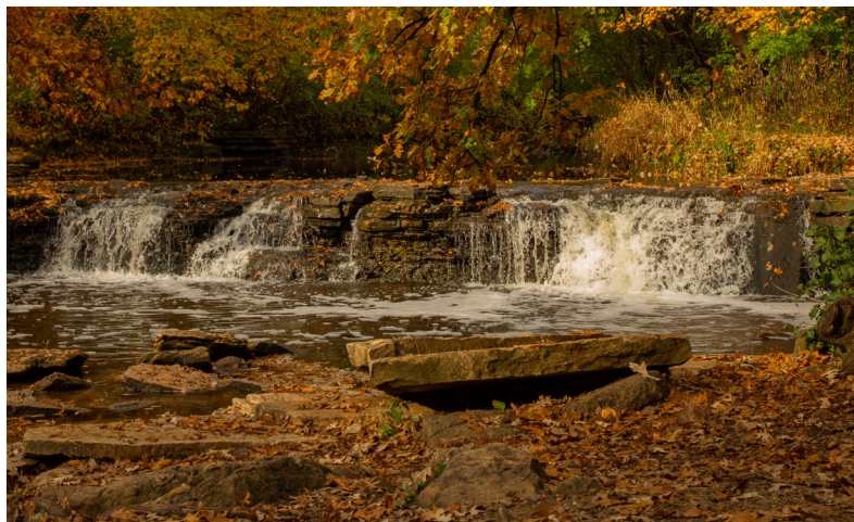
CCC-built Rocky Glen Dam at Waterfall Glen
